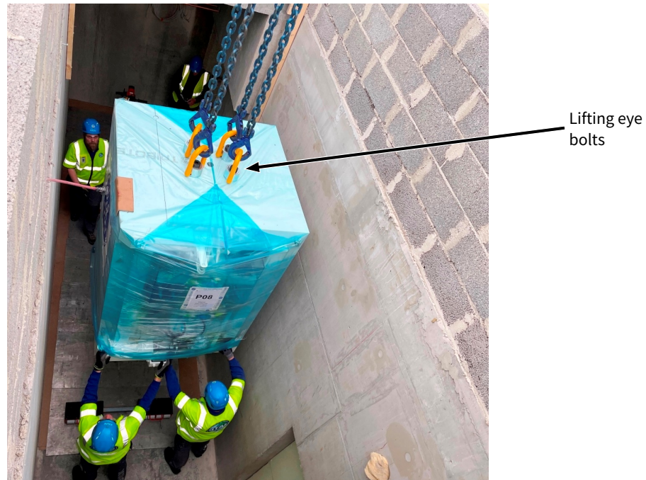
Figure 8-2: Cyclotron magnet with lifting eye bolts
